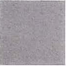
stucco wall finishes darker tone
